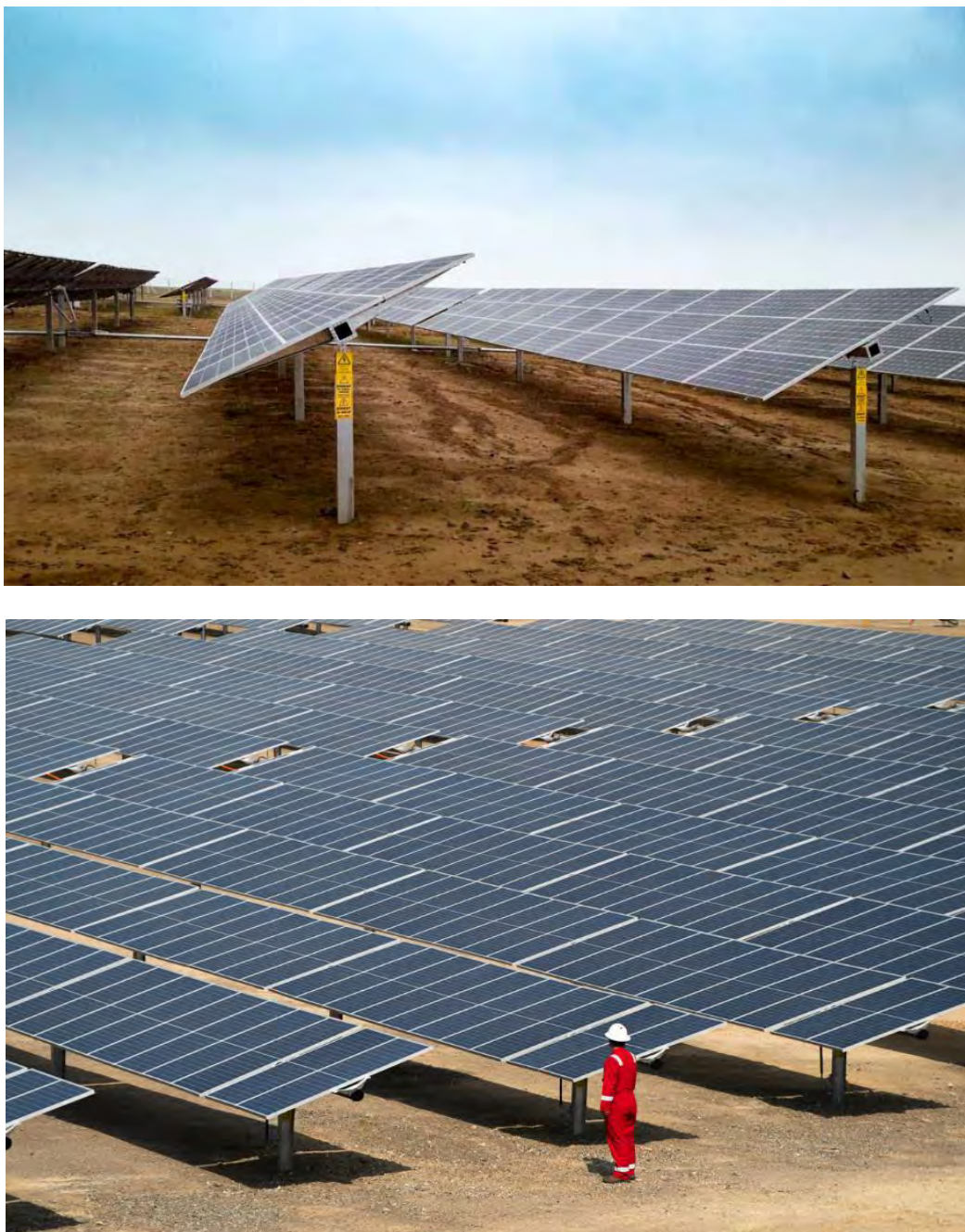
Figure 2-3: Photographs showing Solar Mounting single axis (top) and Solar Modules installed on tables (bottom).
